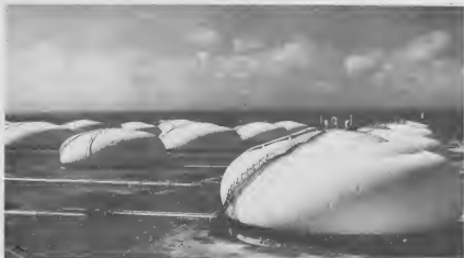
Lago's 100,000-barrel spheroids, covered by literally acres of white paint gleam brightly in the tropical sun.
